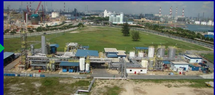
15 MWth Commercial Unit started up in 2011 in Singapore, and operated by Itea until 2013
