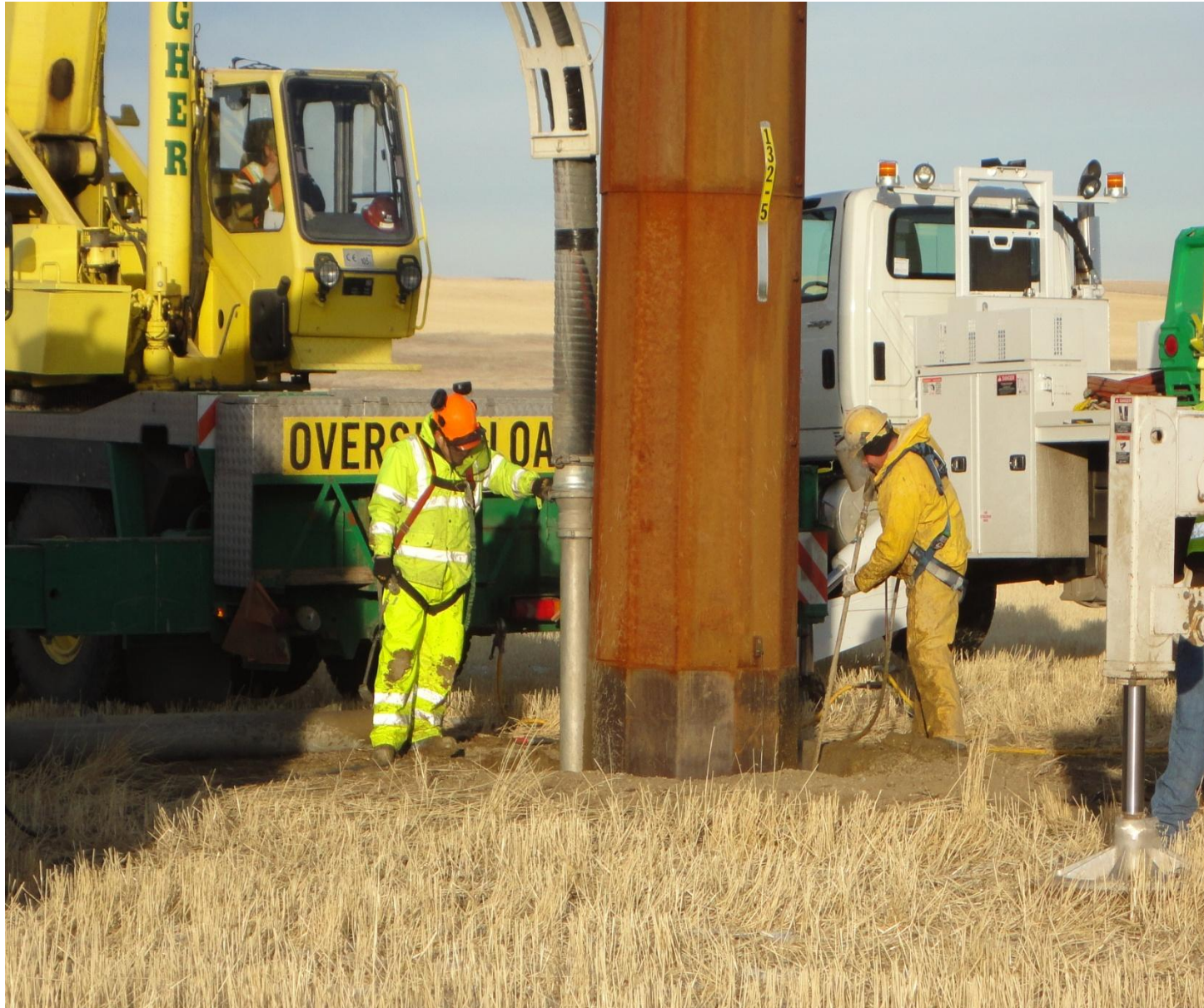
Pole remediation – hydro vac
