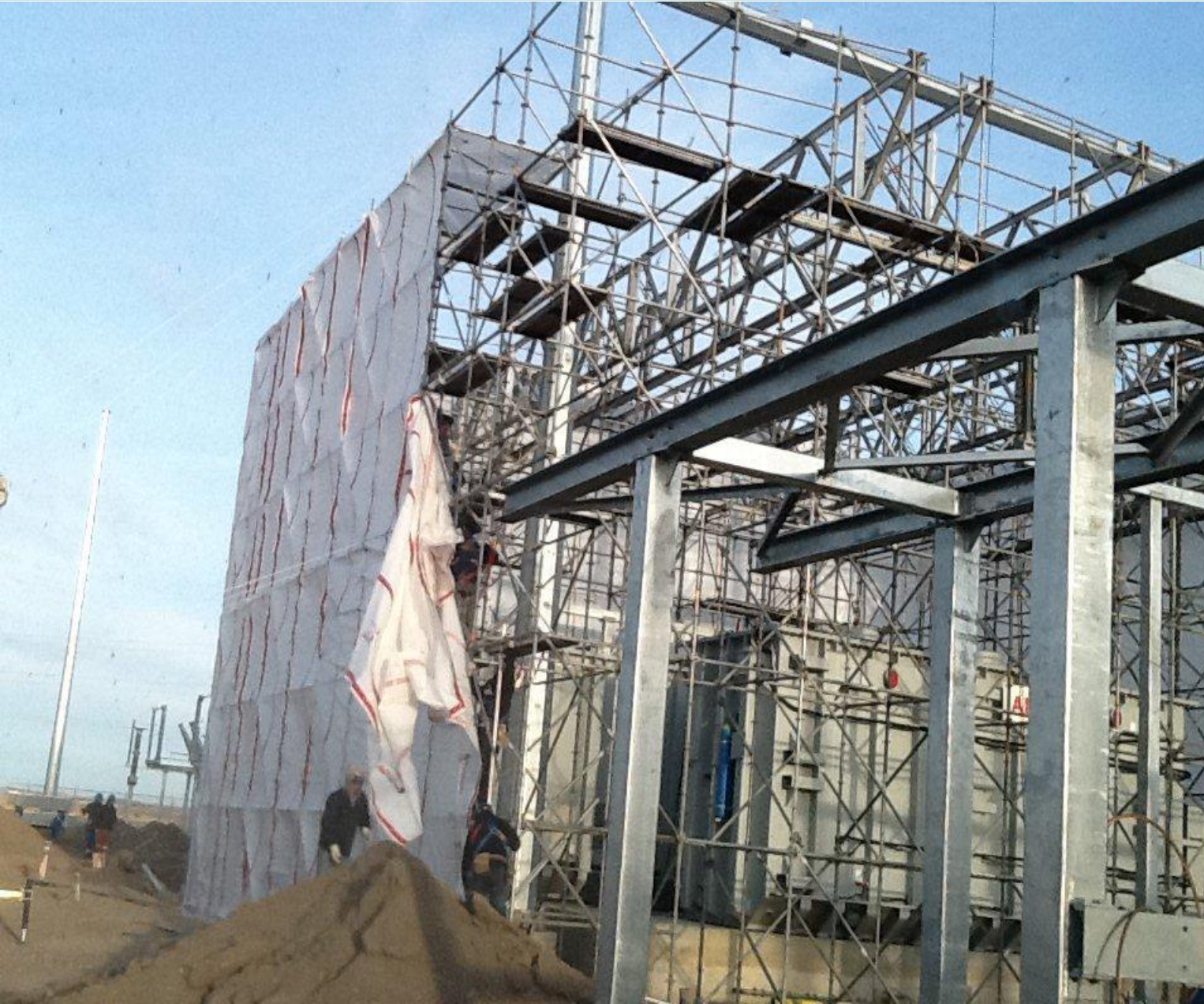
Shelter being built around the PST at 120S substation
